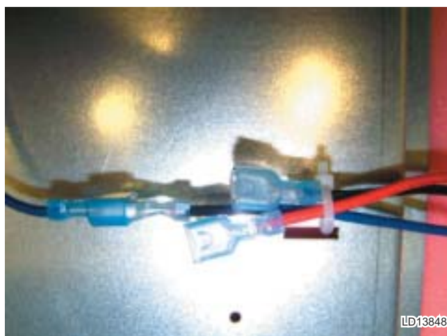
FIGURE 1B - WIRE TO WIRE FAN SPEED SELECTION
